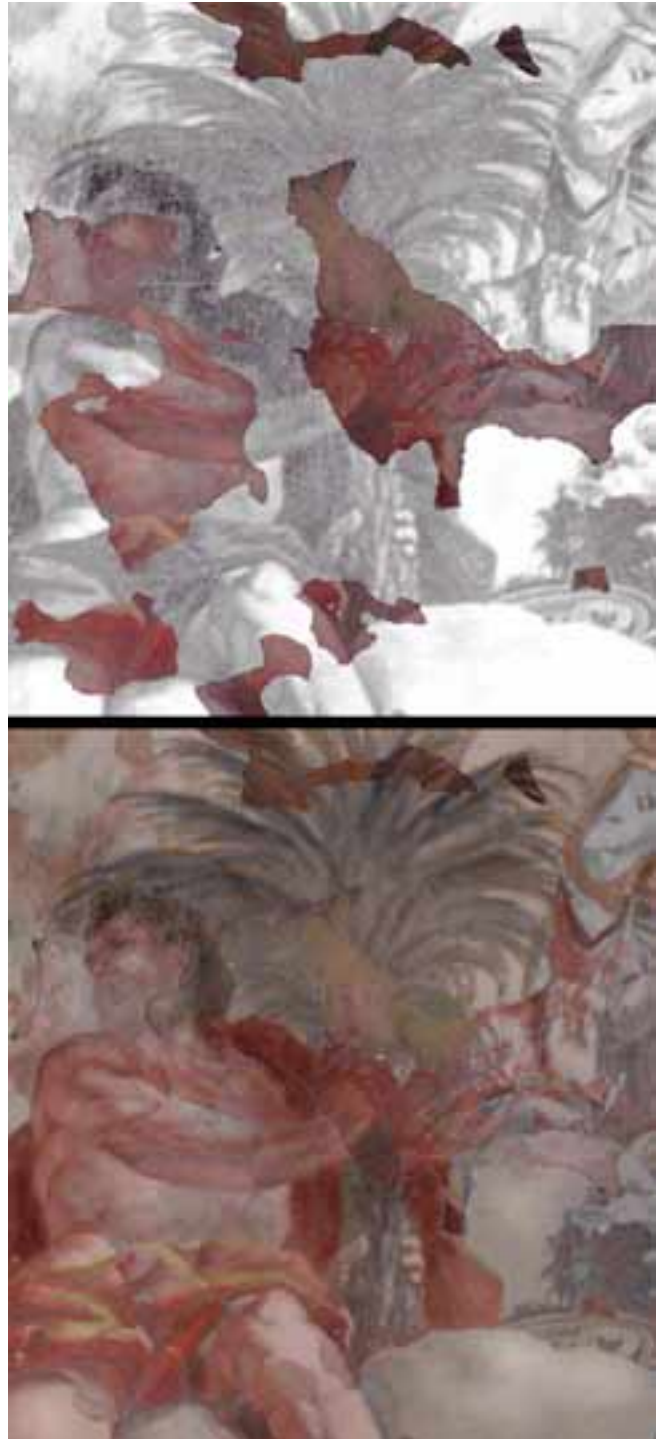
Figure 9. A before and after image of the restoration of the frescoes on the vault of the Santos Juanes Church in Valencia, Spain. Photograph provided by HP in Barcelona.
